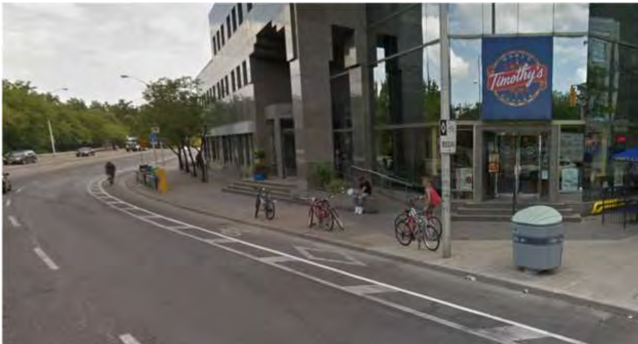
Buffered Bicycle Lane (painted buffer with diagonal hatching)
